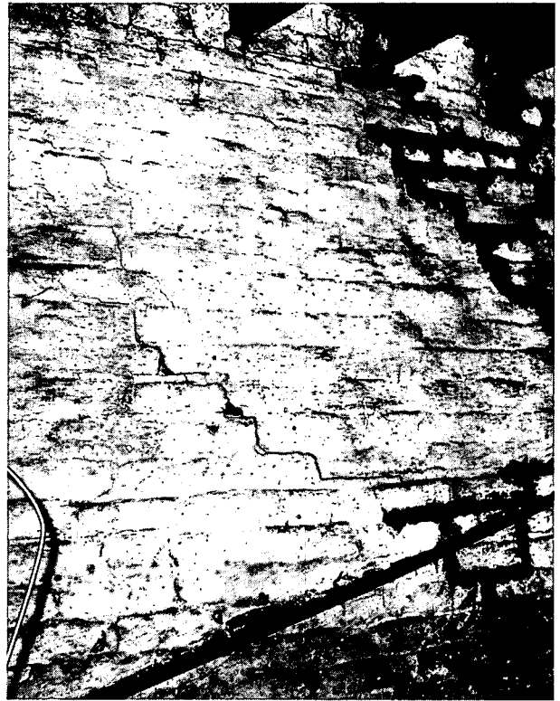
Plate 2 Side wall of Waggon Porch showing extensive cracking
