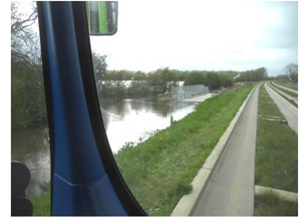
The whole alignment of the Greenway between Swavesey and St Ives is prone to flooding, but the busway itself is generally expected to not flood.
