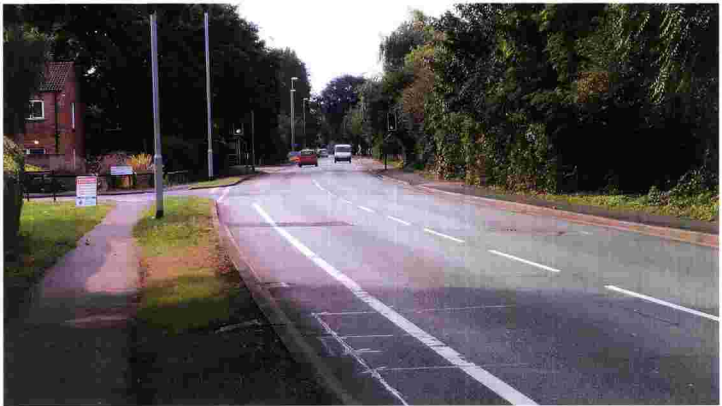
North of Hazelwood Close (Facing South)
