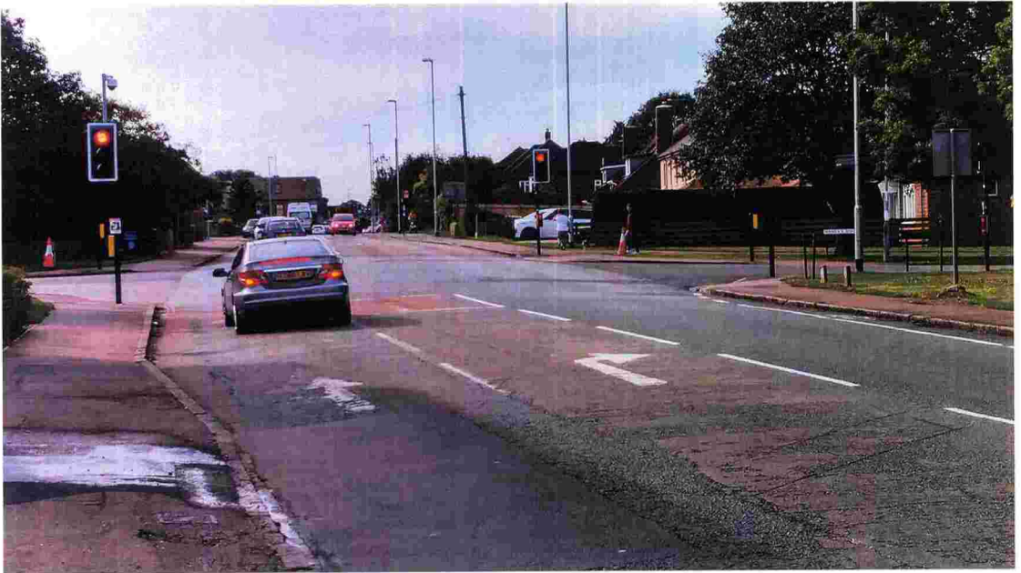
North of Gilbert Road (Facing South)
