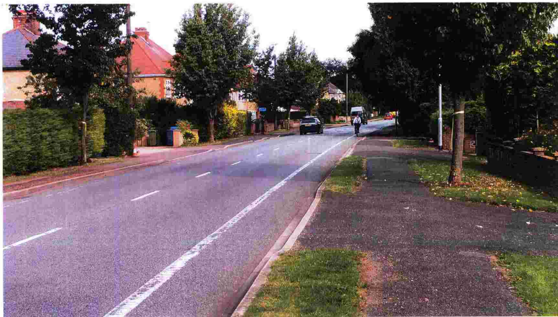
North of Carisbrooke Road (Facing North)
