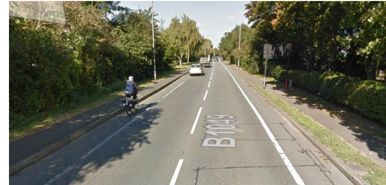
Existing (view north)
