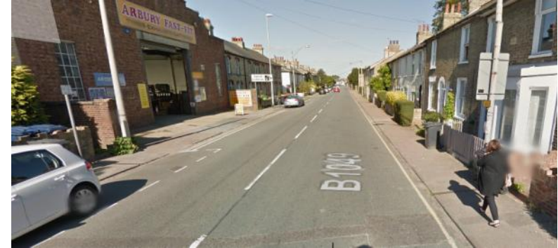
Existing (view north)
