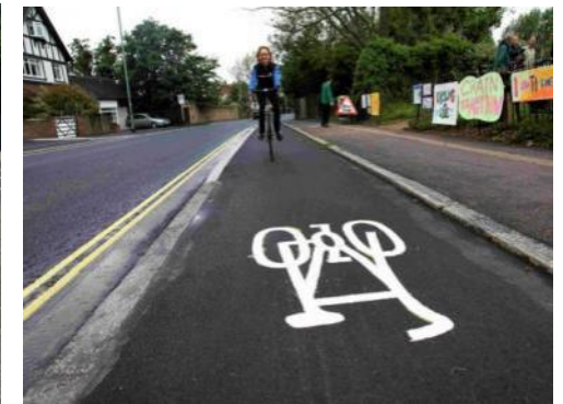
Stepped track ('raised cycleway')
