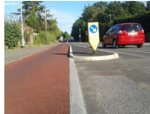
Fully segregated lane/track
