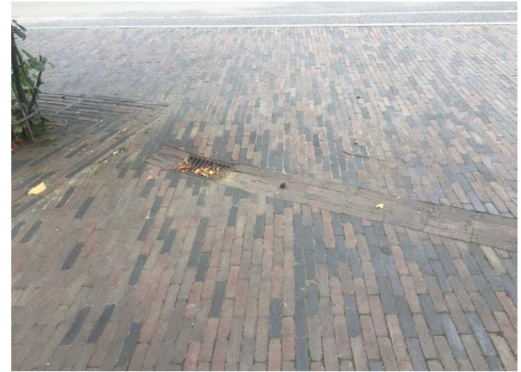
Paving, tree opening and drainage
