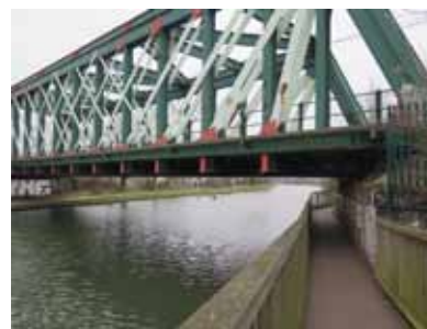
View of narrow link under railway bridge
