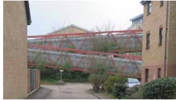
Montage of new ramp to Station Bridge
