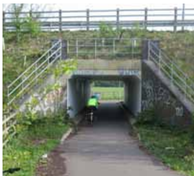
View of new bridge under Long Road
