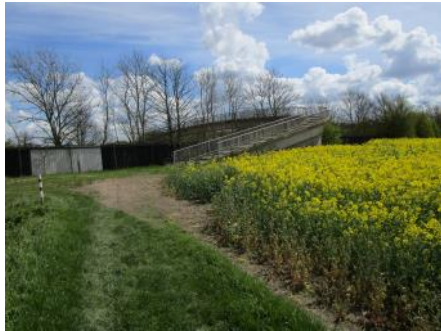
Option iii—The existing bridge showing the stepped ramp.
