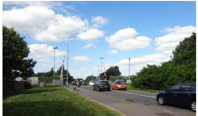
Existing shared cycle path at Yarrow Road level crossing
