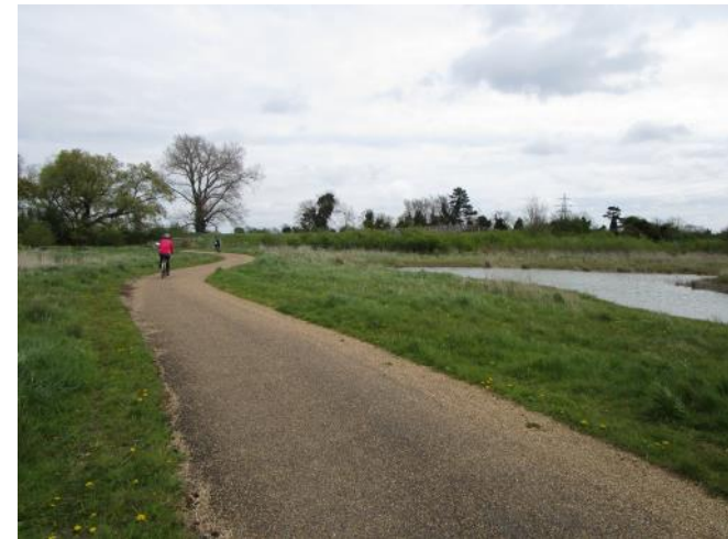
Tar spray and chippings were added to a sealed blacktop surface on this path near Lode.
