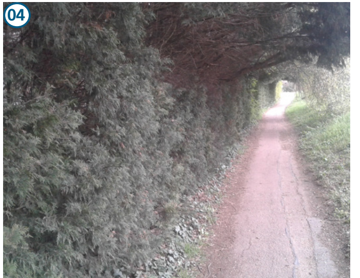
04 Lansdowne Road to Conduit Head Road - looking East Large coniferous hedge and tree planting (TPO Cedar) located along boundary, providing screening for properties. Vegetation will need regularly maintenance and canopy lifted to ensure cyclist are not impeded. Ditch located along boundary. Works maybe with tree Root Protection Areas.
