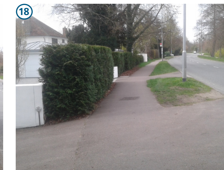
18 Grange Road to Wilberforce Road - looking West Hedges provide screening benefits so should be retained if possible. Verges are of poor quality in places and need treatment / maintenance if retained.
