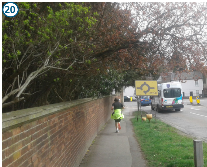
20 Westminster College - looking East Vegetation overhangs footpath and will need to be lifted to allow sufficient height to allow cyclist and pedestrians to move freely.
