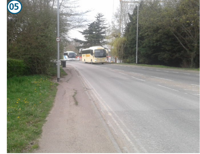
05 JJ Thomson Avenue - looking West Large verges allow room for cycle route with setback hedges providing screening. However, verges narrow and create 'pinch points' at specific locations with likely loss of boundary tree planting and impact on Root Protection Areas
