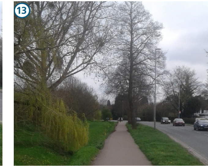
13 Observatory Drive to Storey's Way - looking East Trees in verge to be retained if possible. Offer screening and landscape benefits. Ditch in verge to be realigned to ensure sufficient width and minimise impact on verge tree planting
