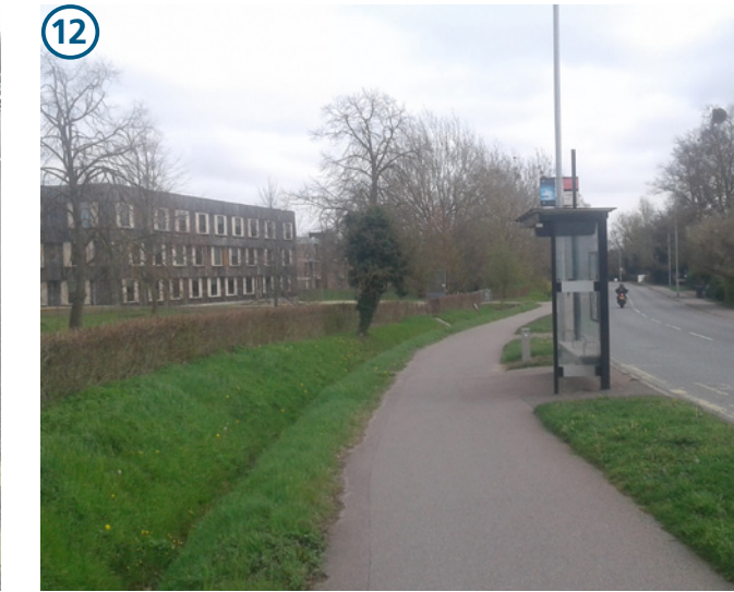
12 Observatory Drive to Storey's Way - looking East Verge to be retained, but requires realignment of ditch to ensure sufficient space for footpath and cycleway. Consideration to location of bus stop required to most suitable position.
