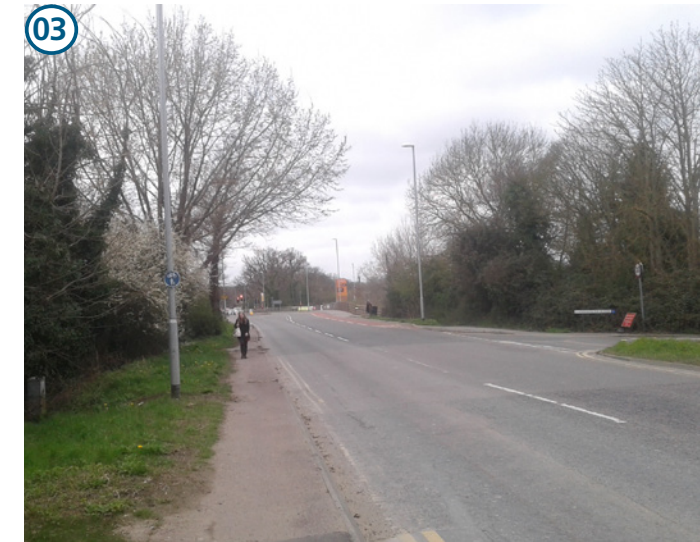
03 Opposite Lansdowne Road - looking West Likely loss of selected mature boundary trees are anticipated. A ditch runs along the boundary and proposed cycle lane will need to consider level change and drainage implications.
