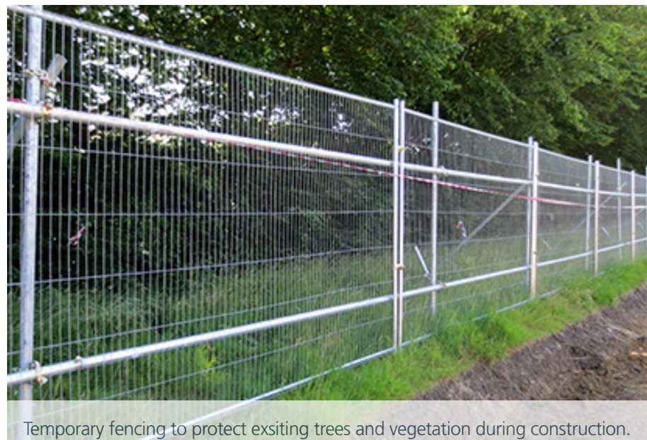
Temporary fencing to protect existing trees and vegetation during construction.
