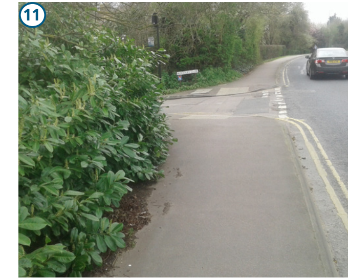
11 Hedgerley Close- looking West Dense vegetation on corner may need to be cut back to improve sight lines near crossing
