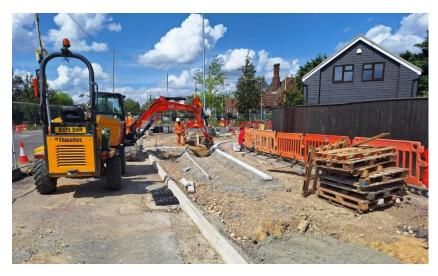
We are currently working on the north-east quadrant of the King's Hedges crossroads, installing a new kerb line and constructing pavements. Once complete, we will start on the south-east quadrant outside the Co-op. This is scheduled to begin in mid-September.
