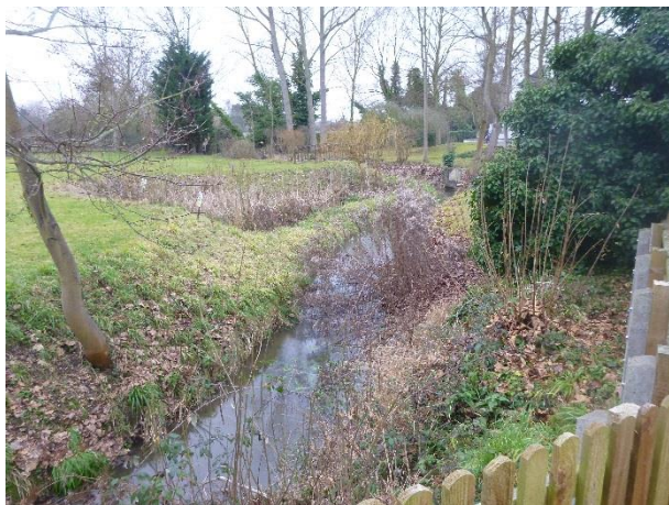
Figure C-3 – Upstream of the culvert under Herschel Road
