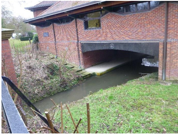
Figure C-1 – Downstream of Sylvester Road bridge
