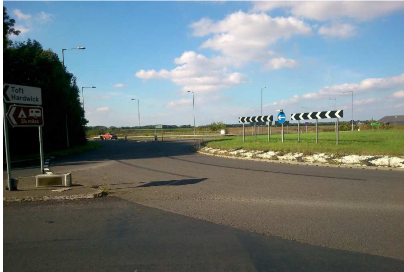
Figure 27 - Hardwick Junction South Roundabout
