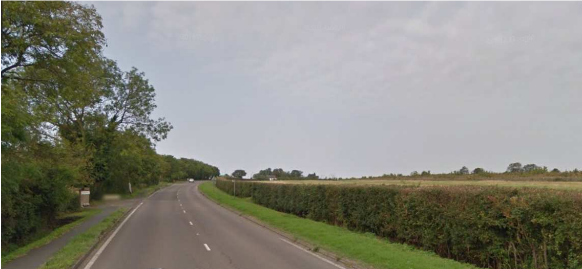
Figure 21 - Bourn Roundabout to Hardwick Junction – looking North West
