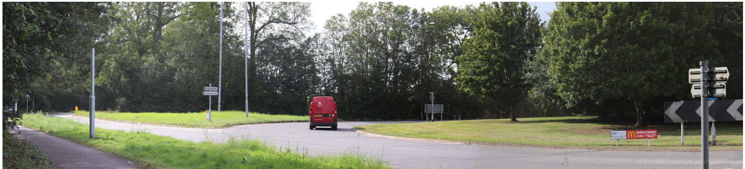
Photograph 7: A1303 roundabout with St Neot's Road, north east of Sector C This viewpoint looks westward, away from Cambridge. Tree belts around the area of Sector C between the A428 and St Neots Road are prominent in the view and prevent wider views. Extensive road infrastructure is visible, but little other built development.
