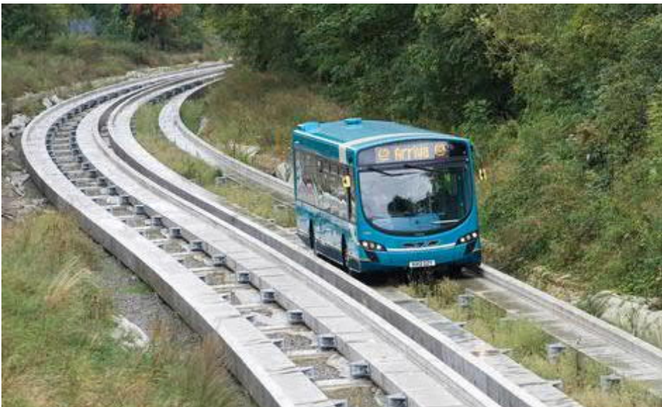
Figure 6.1: Precast kerb guided busways – Luton-Dunstable busway during construction and testing
