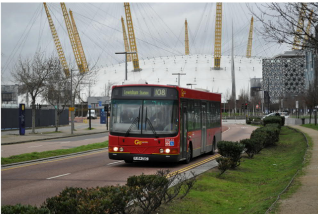
Figure 5.6: Millennium Dome Busway
