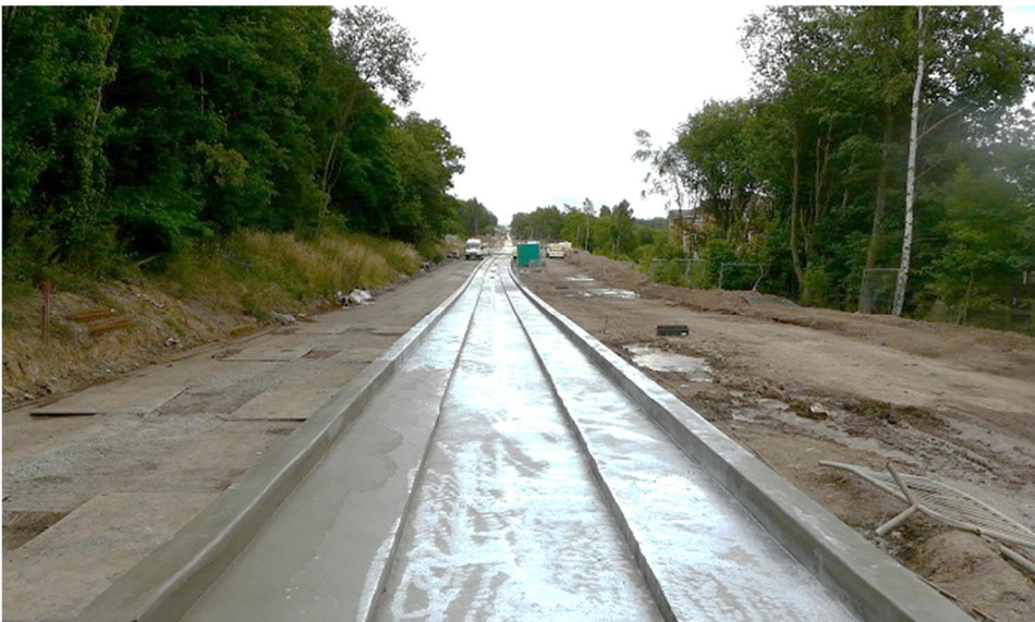
Figure 6.2: Slip formed kerb guided busways – Leigh-Salford-Manchester Bus Rapid Transit scheme during construction
