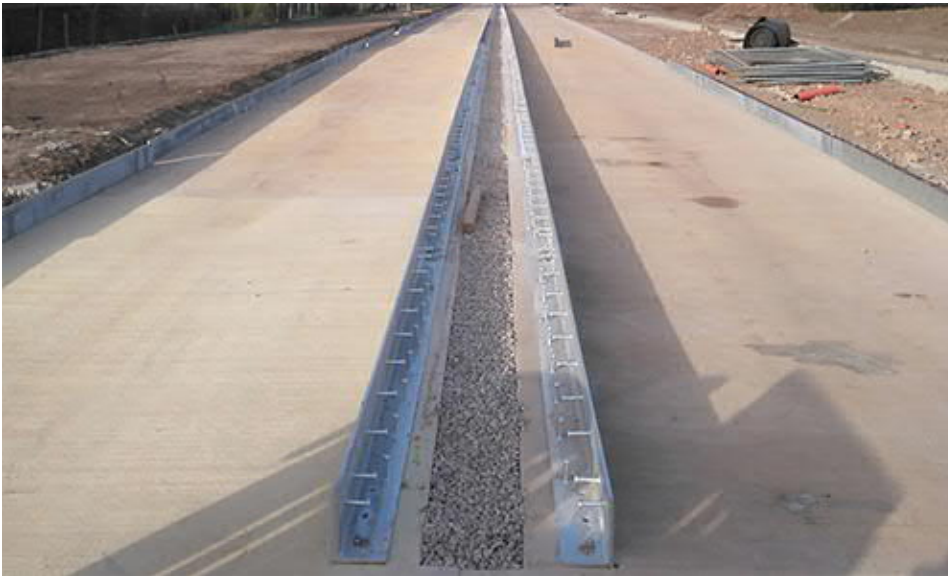
Figure 6.3: CRCP kerb guided busways – Bristol Metrobus during construction
