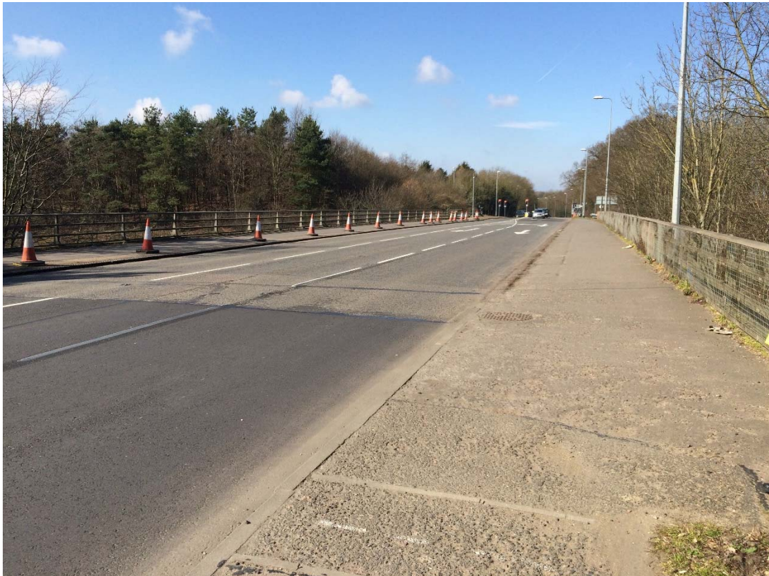
Photo 1 – View Over Rectory Farm Bridge Looking East
