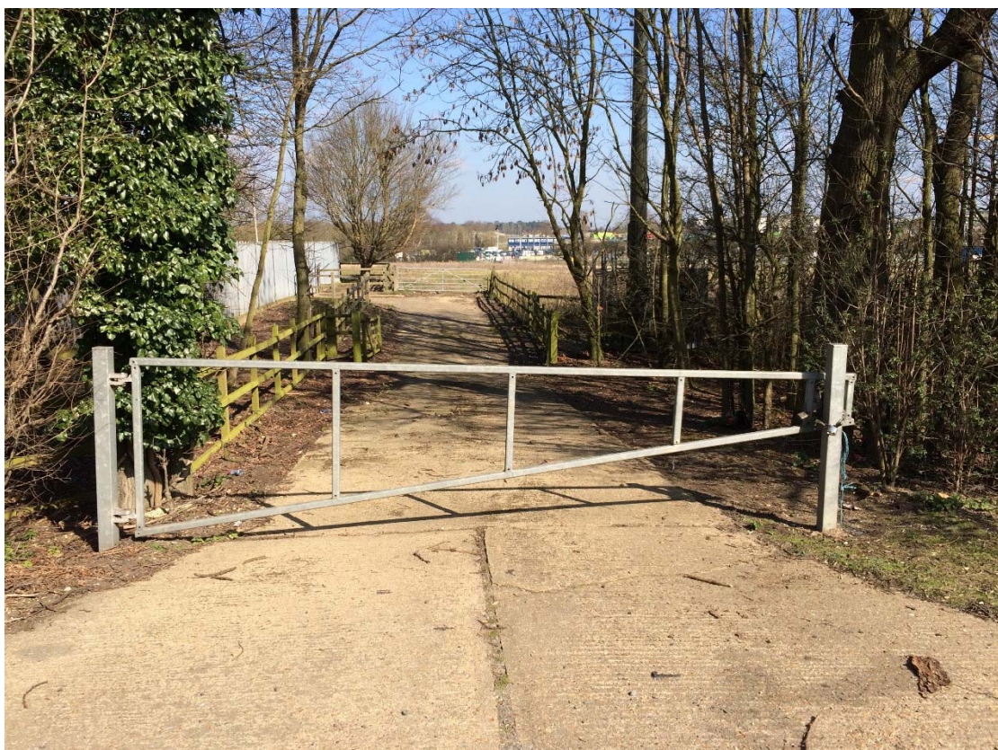
Photo 8 – Access to GVC Approximately 60m North East of Rectory Farm Bridge
