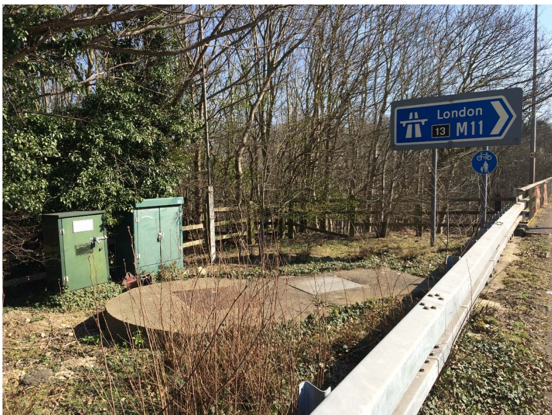
Photo 10 – Utilities with in the North West Verge
