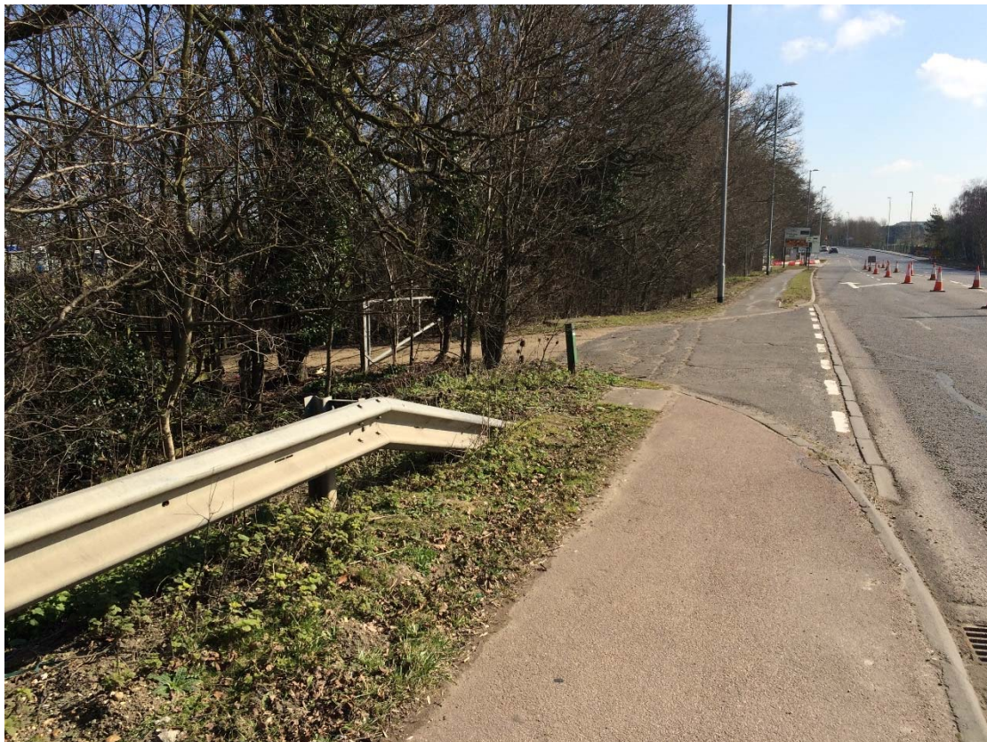
Photo 7 – Access to GVC Approximately 60m North East of Rectory Farm Bridge
