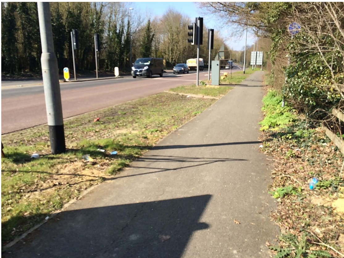
Photo 4 – View of A1303 Traffic Signals at M11 Off-slip Junction
