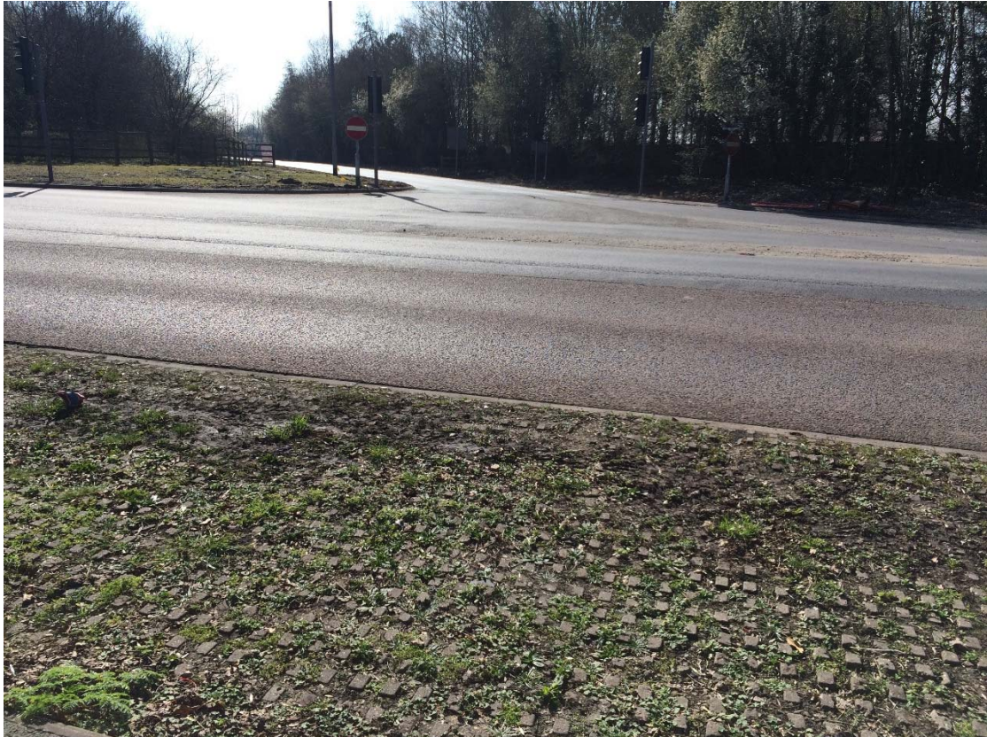
Photo 3 – View of M11 Off-slip Junction
