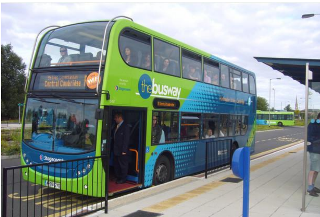
Figure 7-5 Vision to reality: better quality PT on the Guided Busway
