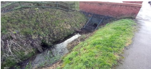
Figure 5.1.1-49 – Grated Culvert
