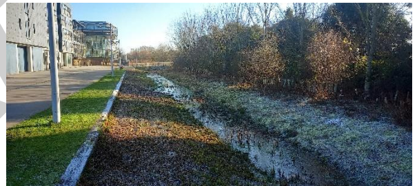
Figure 5.1.1-26 – West Cambridge Canal East 2
