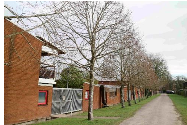
Figure 9-5 – Grade II* listed Clare Hall College complex
