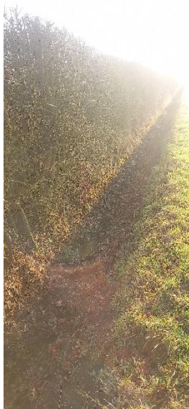
Figure TR5.1.A-69 – Dry Drain
