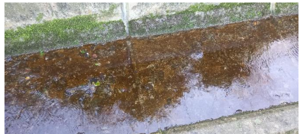
Figure TR5.1.A-14 – Concrete Channel 2
