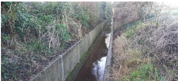
Figure TR5.1.A-11 – Concrete Channel
