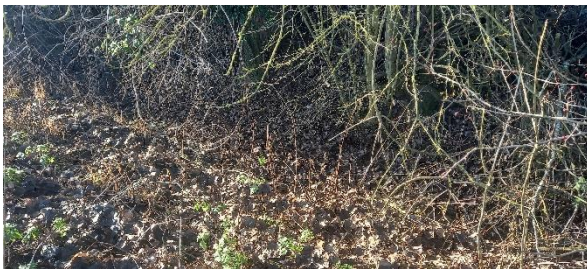
Figure TR5.1.A-65 – Dry Ditch
