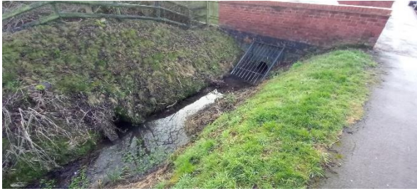
Figure TR5.1.A-49 – Grated Culvert
