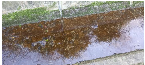
Figure TR5.1.A-12 – Concrete Channel 2
