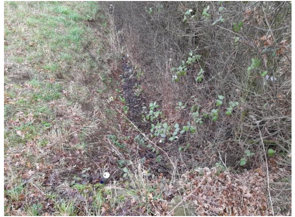
Figure TR5.1.A-74 – Dry Ditch
