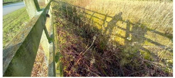
Figure TR5.1.A-62 – Dry Ditch
