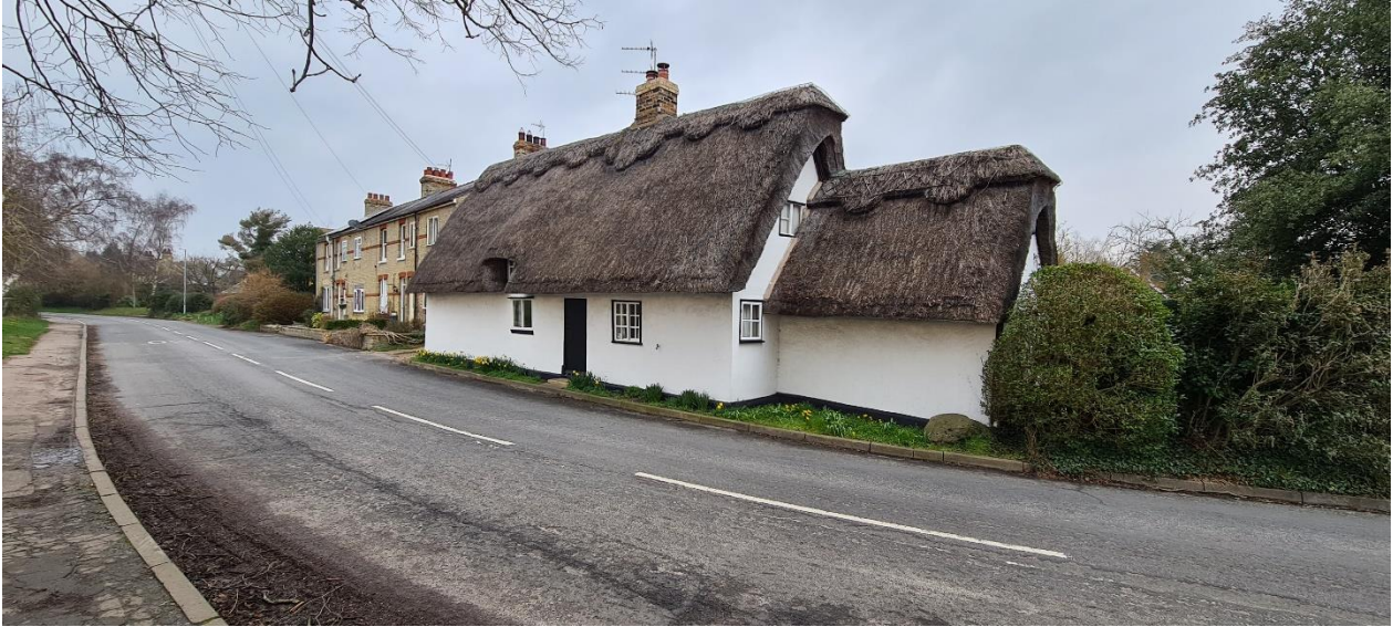
Plate TR7-6-9 - Cottage at 12, High Street, viewed facing north
