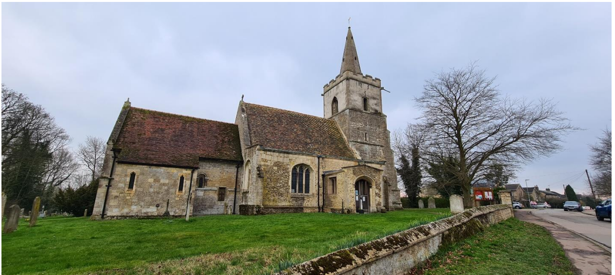
Plate TR7-6-5 - Church of St Peter, viewed facing south-west
