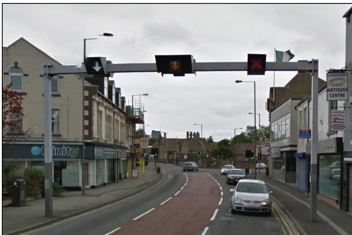
Figure 4: Northbound view of A61 London Road
