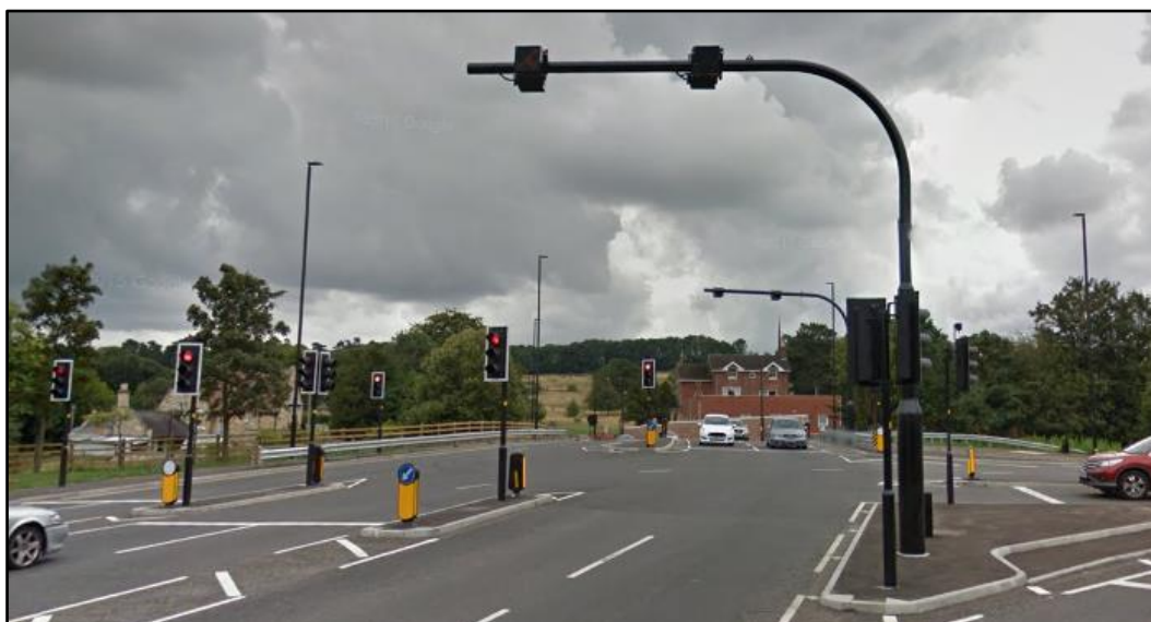
Figure 3: Southbound view of A15 Canwick Road
