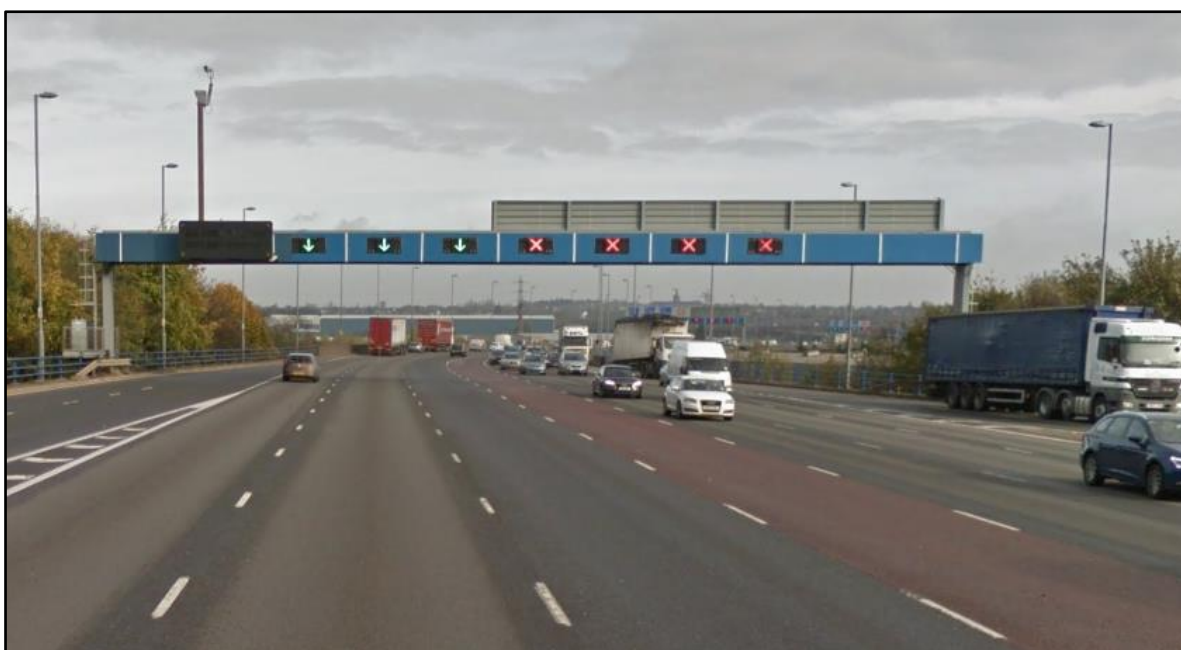
Figure 1: Northbound view of A38(M) Aston Expressway
