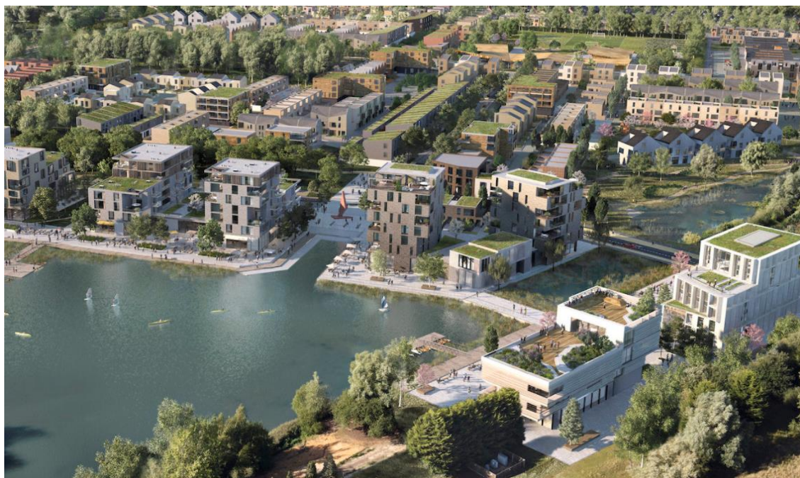
Figure 3.3: Waterbeach Barracks development
