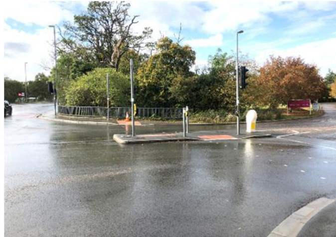
Figure Error! No text of specified style in document.-3: W2 proposed location, a copse at the front of the Park & Ride viewed from the east.
