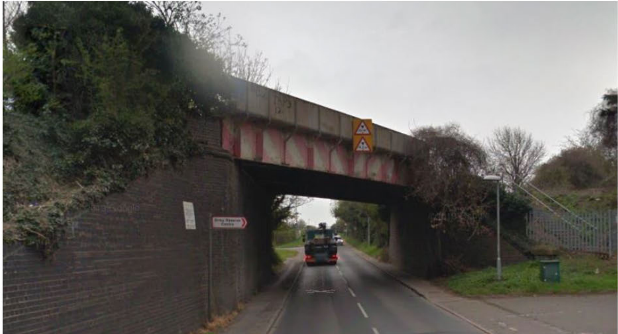
Figure 2: Railway bridge over Coldhams Lane
