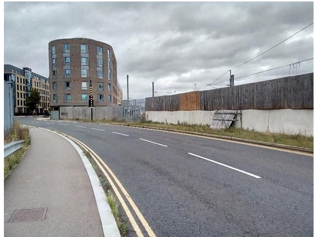
Figure 2.7: Busway, South of Cambridge Station
