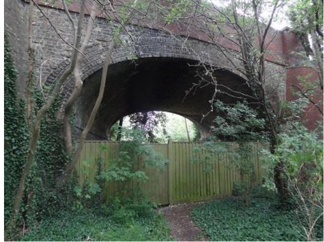
Figure 2.9: Cambridge Road (A1301) Former Rail Bridge
