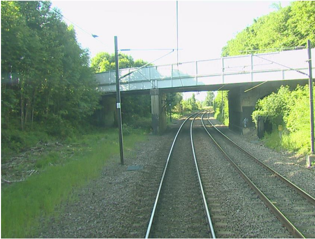
Figure 2.8: London Road (A1301) Rail Bridge
