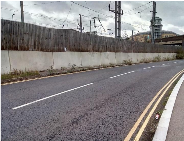
Figure 2.6: Busway, South of Cambridge Station
