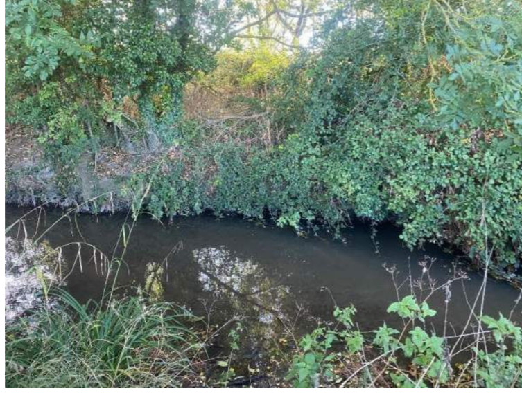
Photograph 15: Typical section of D1 (subreach 2)
