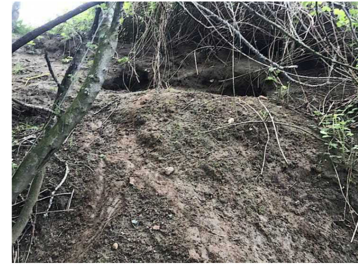
Photo 3. Extensive area of holes on south bank of ditch.
