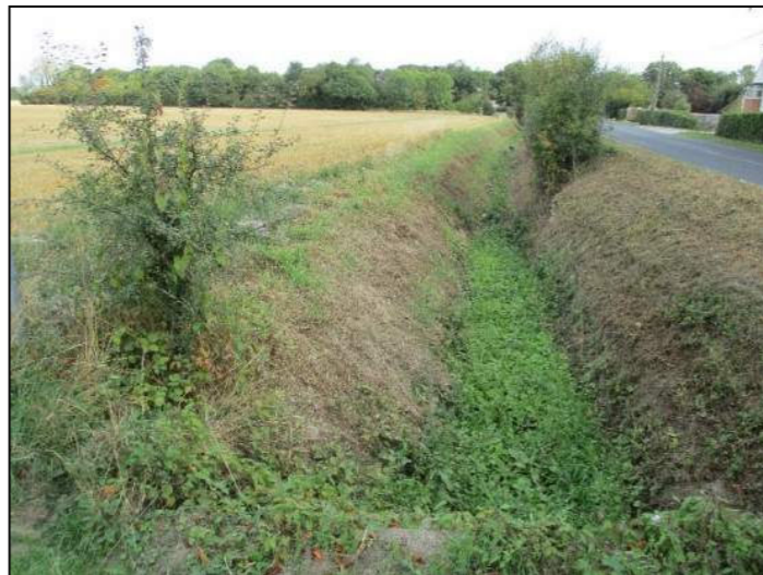
Photograph 12 - Ditch along Granham's Road (W22)
