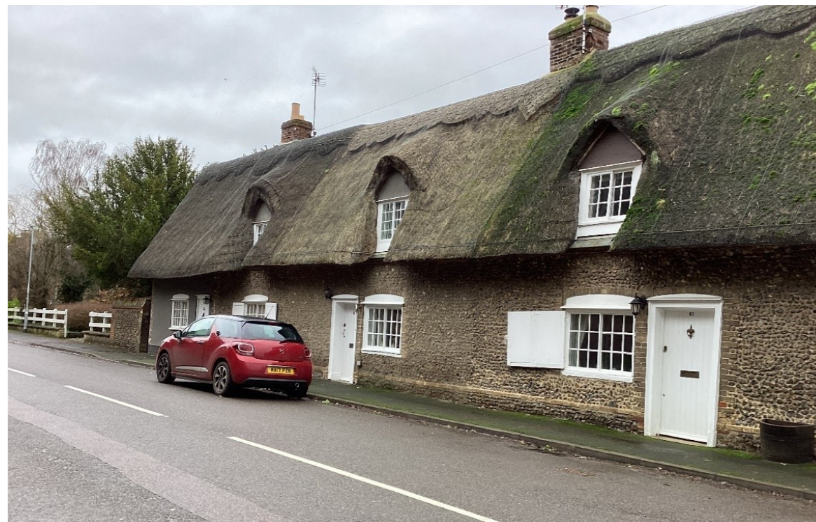
Figure A12.2.7 39 and 41 High Street
