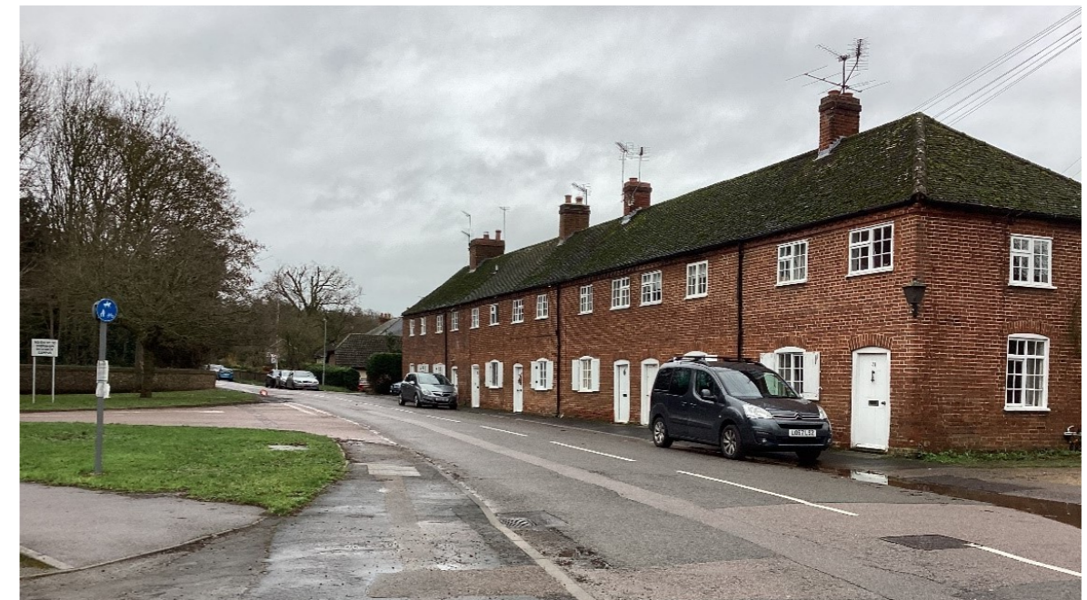
Figure A12.2.8 Brick Row
