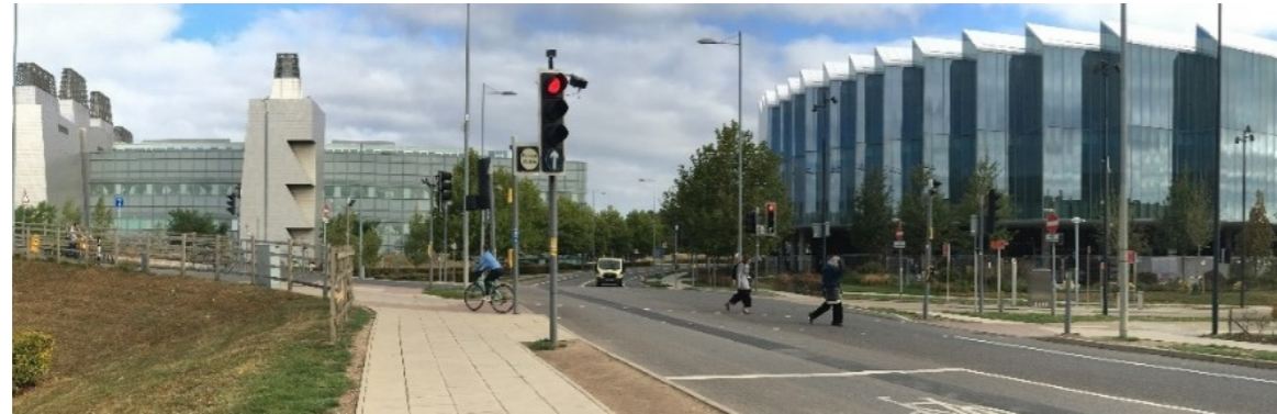
Northern end of Francis Crick Avenue showing the signalised crossroad junction with the existing guided bus way.
