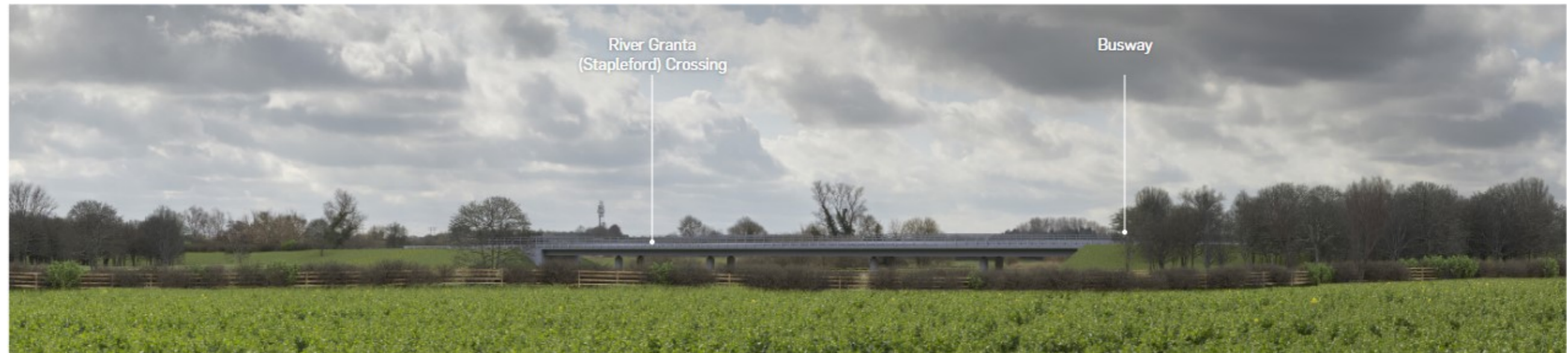
River Granta crossing at Stapleford
