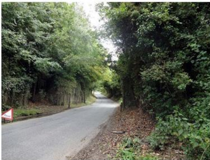
View south-west, showing abutments
