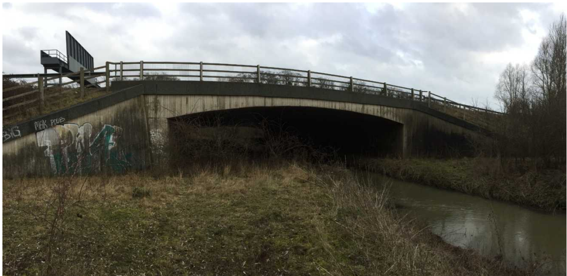
Photo 6-2 A11 River Granta Underpass (West elevation)
