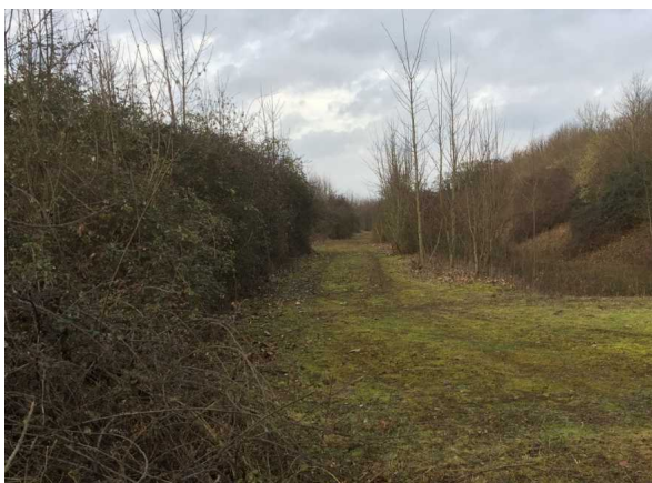
Photo 6-5 A11 East side maintenance track
