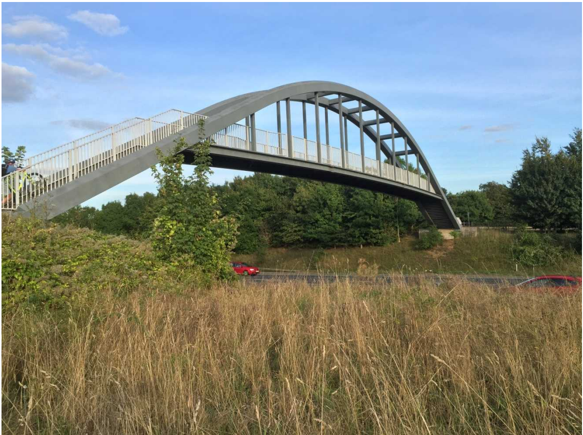
Photo 6-1 A11 Existing Stepped Footbridge.
