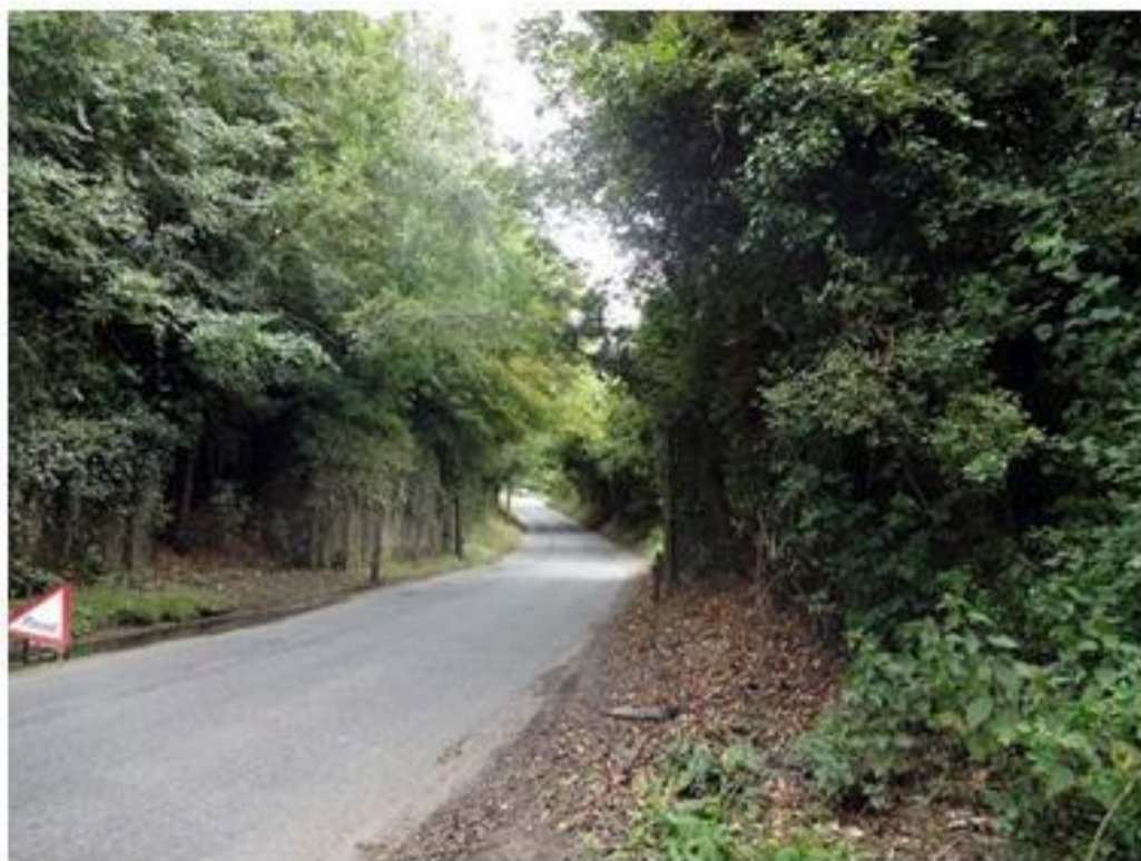
View south-west, showing abutments
