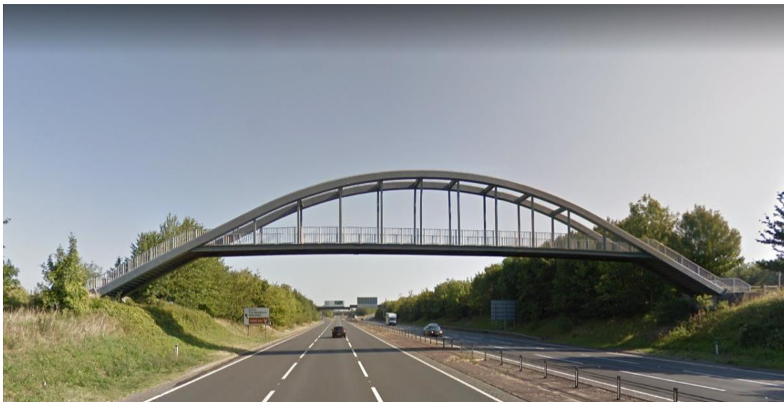
Figure 12.16: A11 Pedestrian Footbridge
