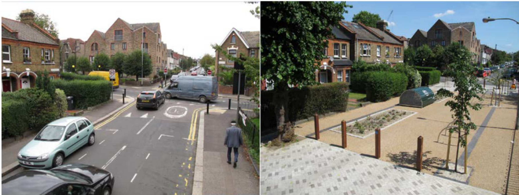
Figure 5.26 Example of a filtered permeability scheme at a junction in Blackhorse Village, Waltham Forest – before and after.
